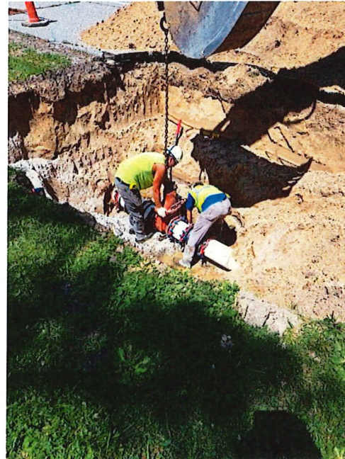
Figure 7 New Flow Meter at LS #2
