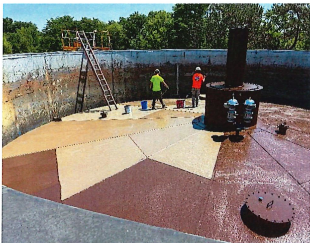
Figure 2 Painting to Protect Digester Cover
