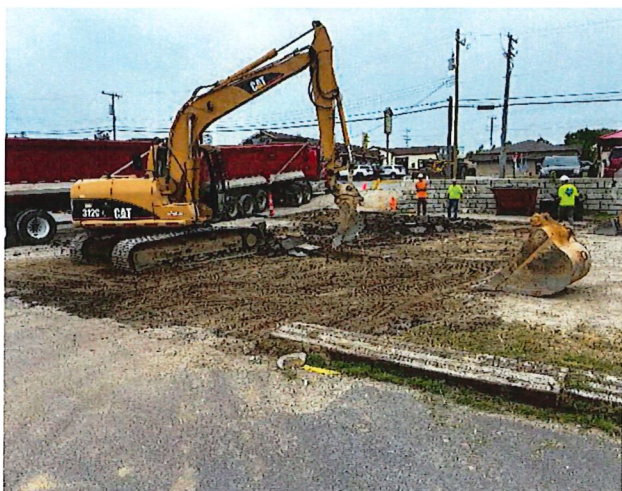
Figure 1 Removal and Backfill of former LS #8
