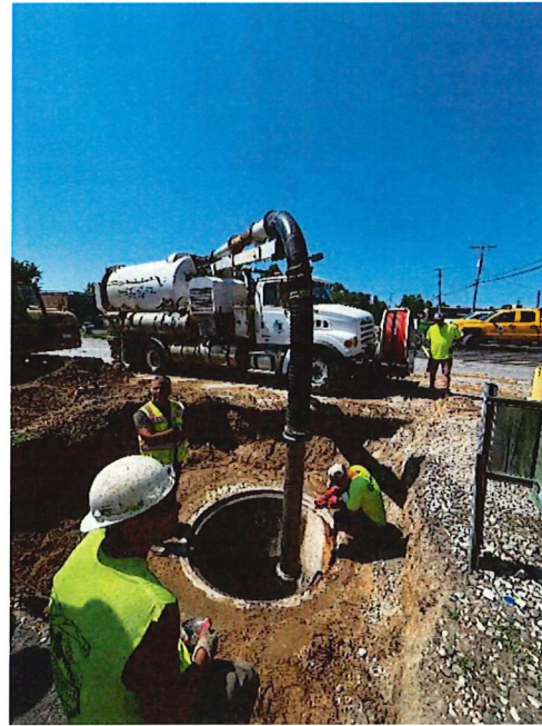
Figure 6 Backfilling Old LS #8
