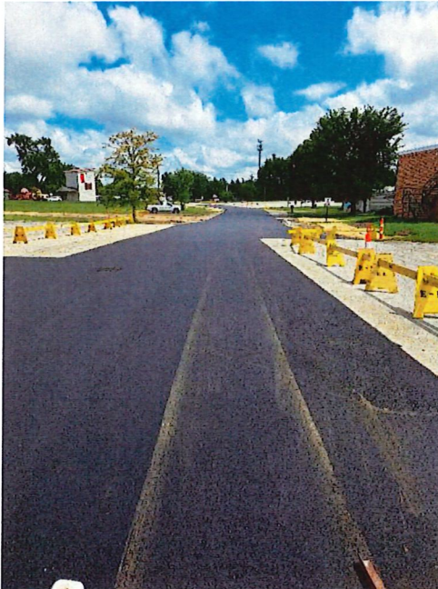
Figure 5 New Park Drive Paving
